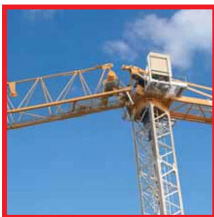
Montaggio del braccio e collegamento al portaralla. Jib assembling and junction to the slewing group.
